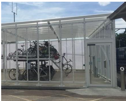
A secure cycle storage hub at Horsham
