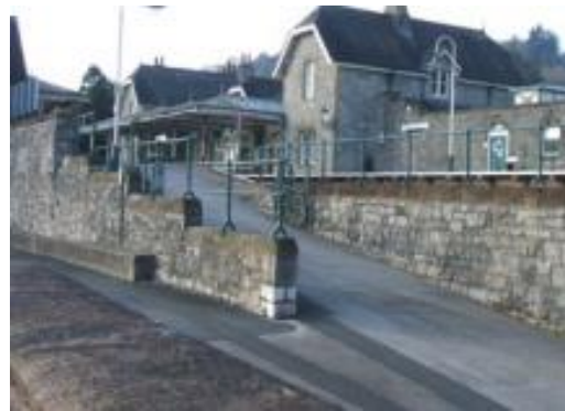
Ramped access to Grange over Sands station, Lake District
