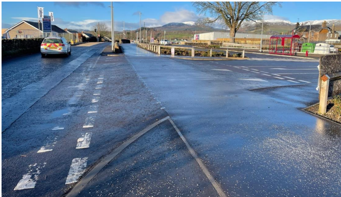
Figure 18 Use of double give way markings and a raised continuous footway on the route to a primary and secondary school on Broich Road in Crieff © Perth & Kinross Council
