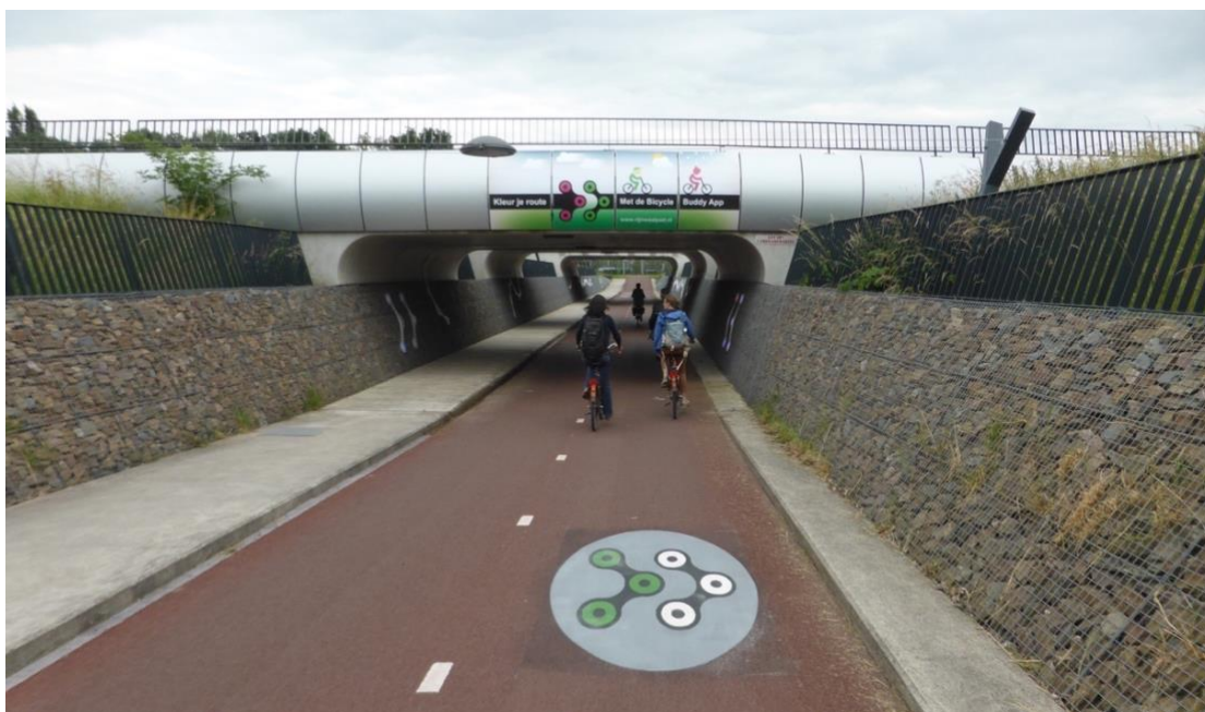
Figure 44 A semi-submerged tunnel under an A-road on a national cycle route in the Netherlands. The retaining walls are designed open outwards to allow for lots of natural light and clear sight lines to the far side © Interreg North-West Europe CHIPS
