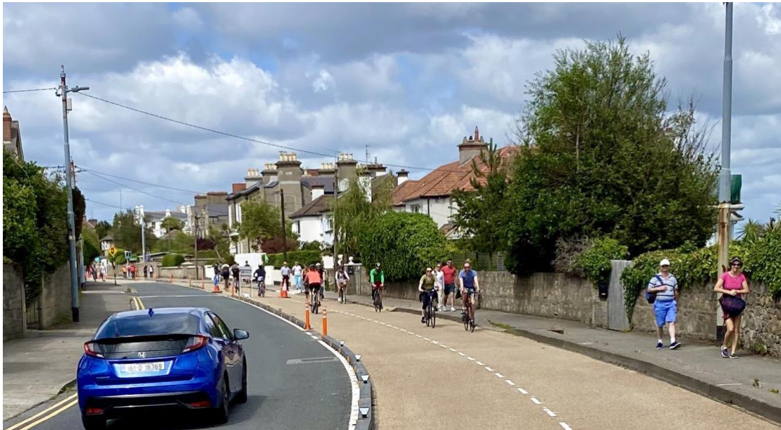
Figure 27 A one-way motorised traffic loop allows the conversion of a motorised vehicle lane into a separated bi-directional cycle track in Rathdown, Ireland © Paul Ohara
