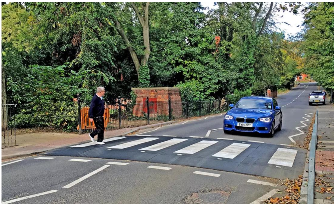
Figure 20 Example of a temporary raised level zebra crossing © Rosehill Highways
