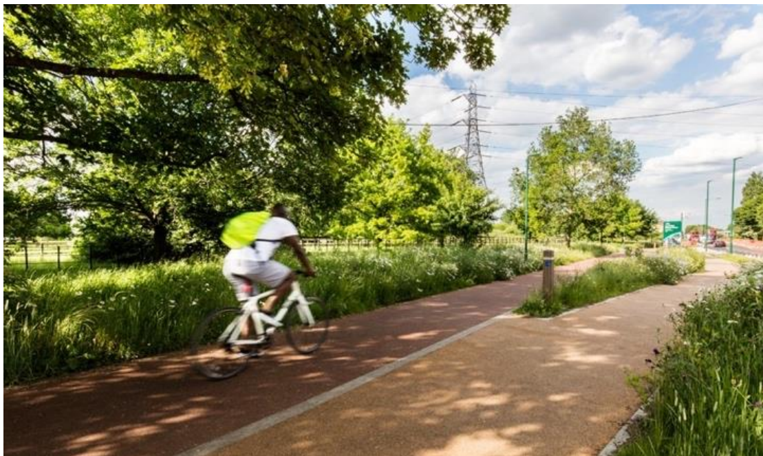
Figure 43 Lea Bridge Road, Mini Holland, segregation between walking and cycling is fundamental to future-proof for the uptake of ecycling. Designing for inclusive cycling as standard is as important in rural areas as in urban areas © Photography: Alexander Christie, Scheme Design: LBWF Highways and what if: projects
