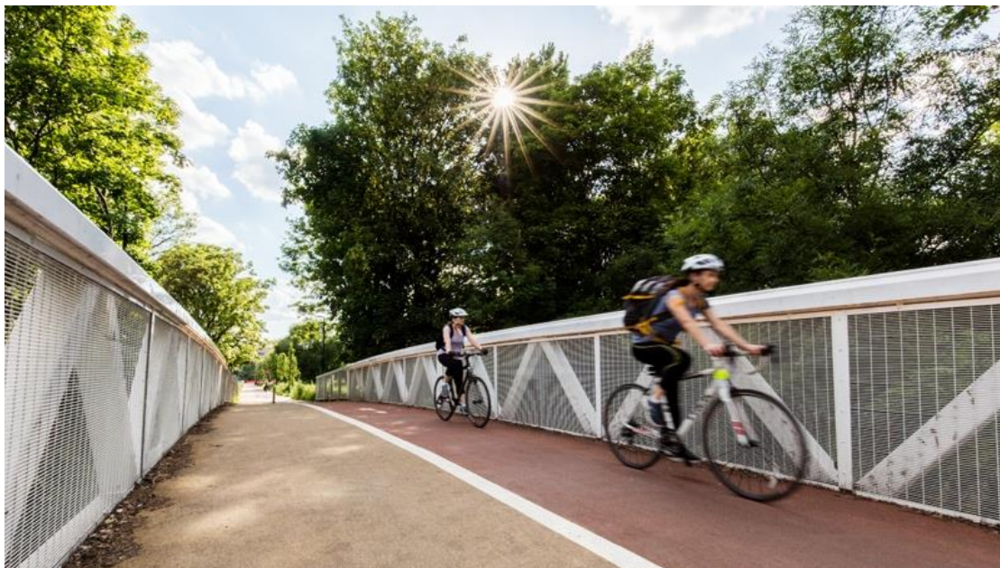
Figure 29 Separated walking and cycling bridge, Lea Bridge Road in Mini Holland © Photography: Alexander Christie, Scheme Design: LBWF Highways and what if: projects
