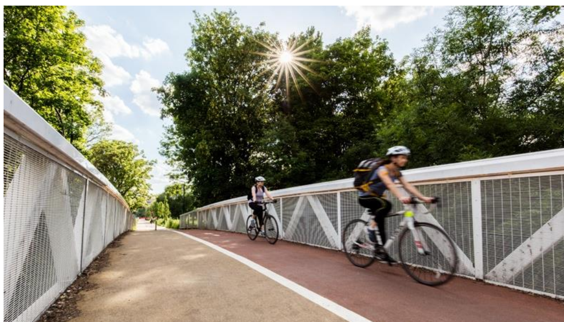
Figure 1 A world class separated walking and cycling bridge, Lea Bridge Road in Mini Holland, © Photography: Alexander Christie, Scheme Design: LBWF Highways and what if: projects
