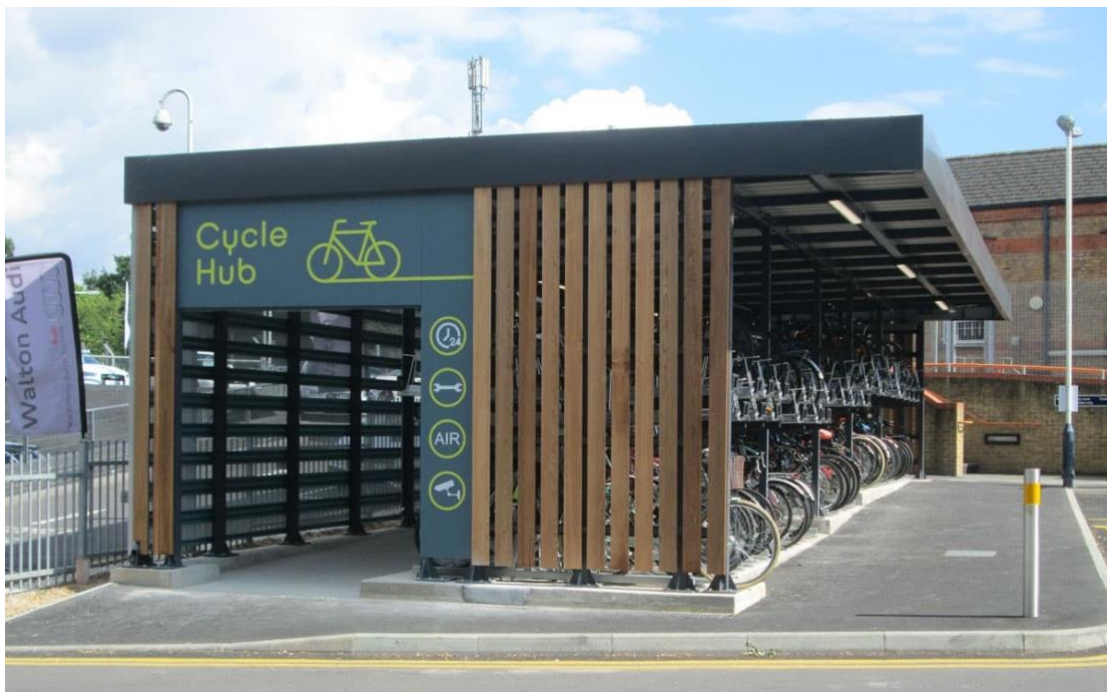
Figure 35 A mobility hub with space for 150 cycles, CCTV and lighting and convenient to the local train station © Cyclepods Ltd
