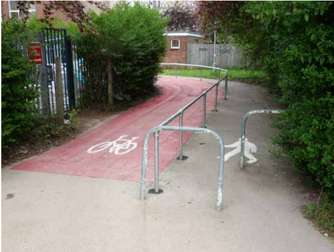
Figure 7.4 Shared use segregated by barrier
