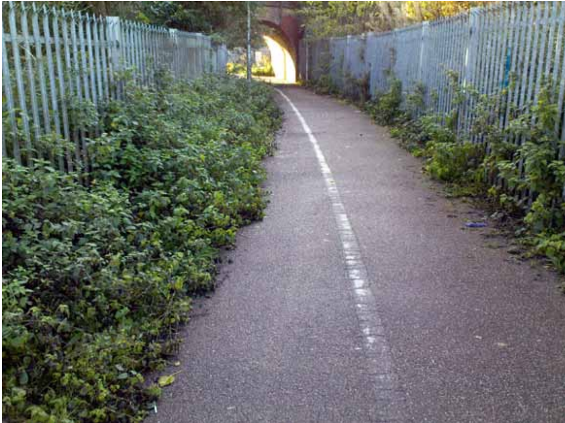
Figure 6.7 Unchecked growth of vegetation leading to a reduced level of service
