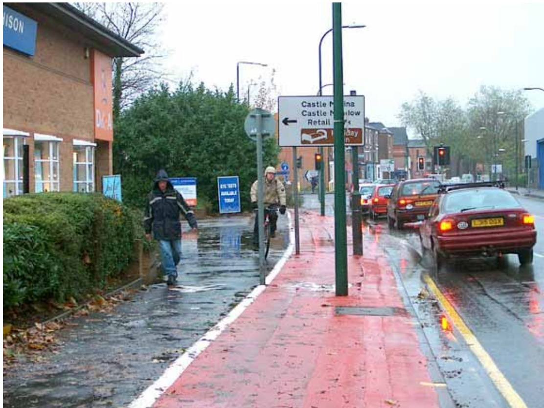
Figure 6.6 Posts obstructing a shared use route
