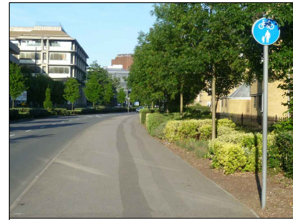
EXAMPLE OF SHARED USE CYCLE PATH No segregation between cyclists and pedestrians.
