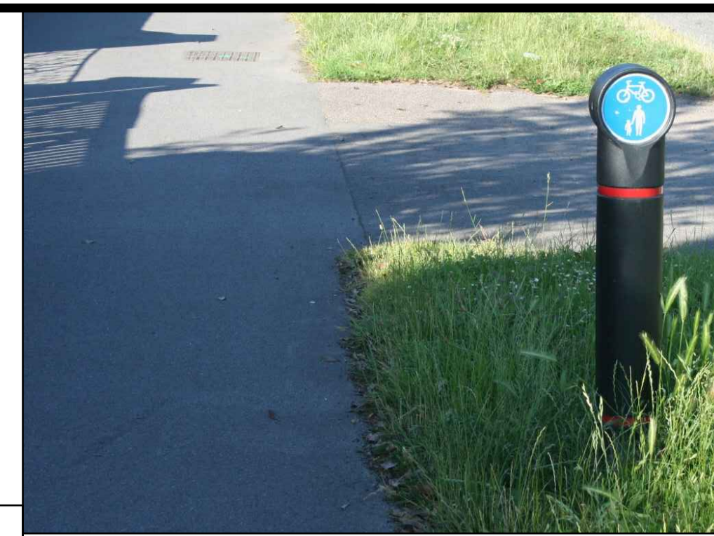
EXAMPLE OF CYCLE PATH BOLLARD Shows shared use cycle path (may show segregated cycle path instead).
