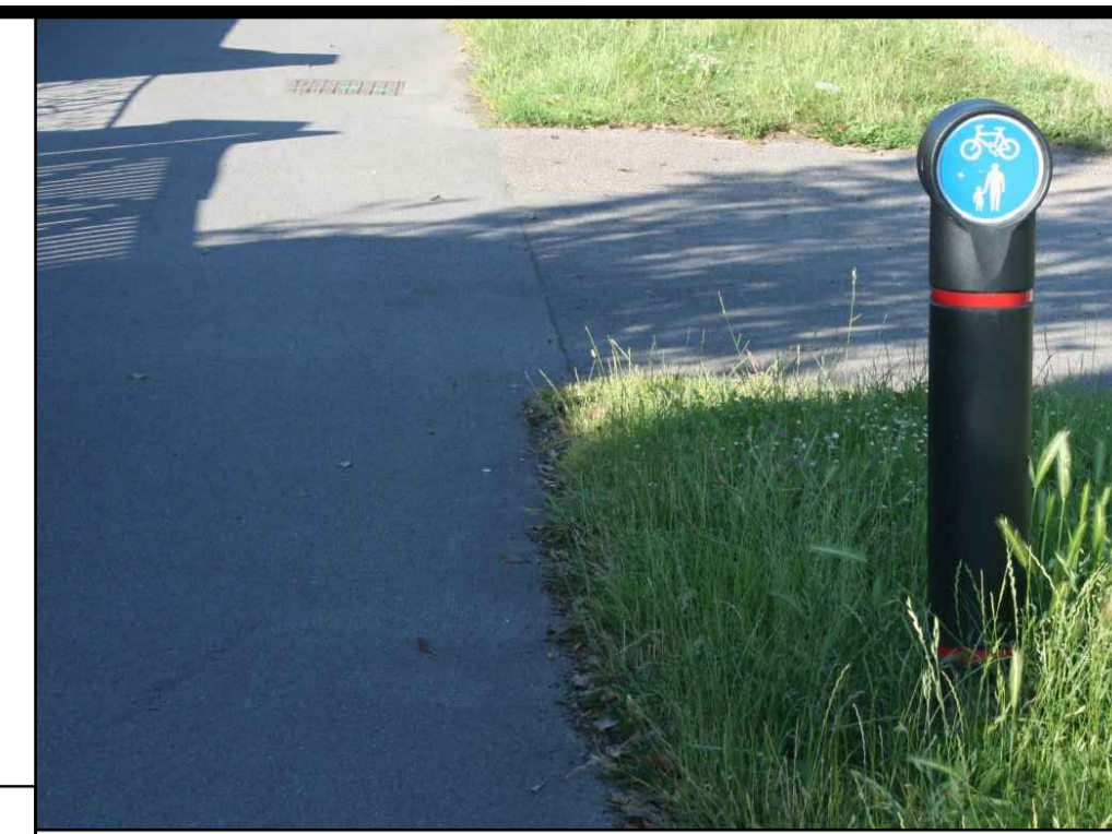
EXAMPLE OF CYCLE PATH BOLLARD Shows shared use cycle path (may show segregated cycle path instead).
